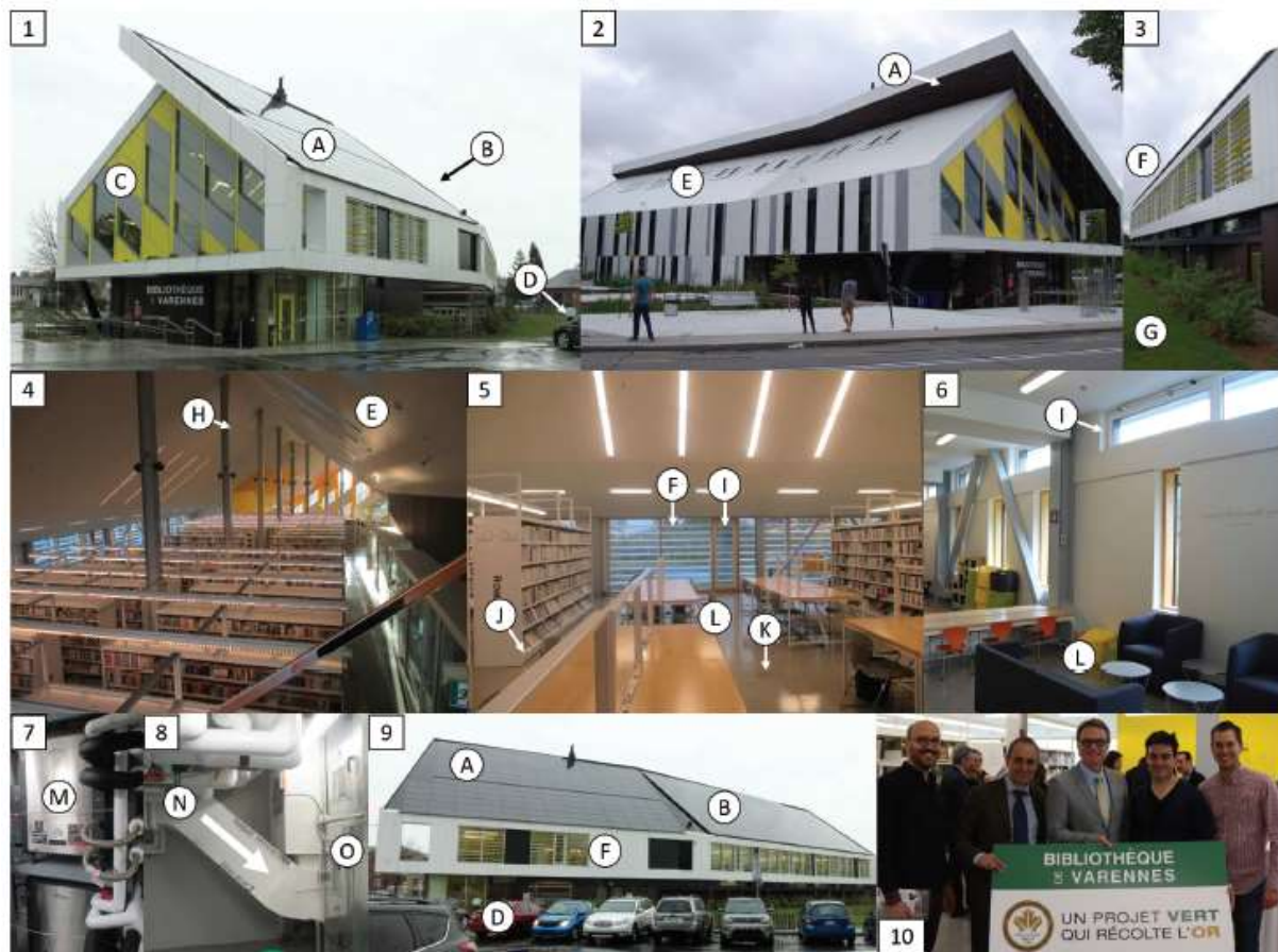
Figure 15: Varennes Library tagged images. (1) entrance, southwest view; (2) north façade; (3) south façade; (4) second floor, facing west; (5) second floor middle section, facing south; (6) ground floor facing south; (7-8) mechanical room; (9) south façade; (10) official opening ceremony, from left to right: Dr. Konstantinos (Costa) Kapsis, Dr. Andreas K. Athienitis, Major Martin Damphouse, Vasken Dermadiros and Remi Dumoulin. (A) forced convected BIPV and BIPV/T area; (B) naturally converted BIPV portion (out of view); (C) west façade, vine supports; (D) two car charging station; (E) skylights on norther roof; (F) fixed exterior louvers, solar shading; (G) geothermal boreholes; (H) ceiling fans; (I) motorized windows; (J) displacement ventilation integrated to bookshelves/stacks; (K) underfloor ventilation diffuser; (L) hydronic radiant slab; (M) geothermal heat pumps; (N) BIPV/T heat into air-handling unit(AHU); (O) AHU. (Dermadiros et al. 2019)
