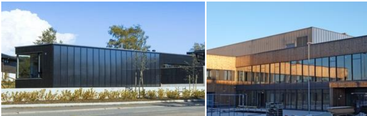
Figure 8. Facade-integrated AventaSolar collectors: installations in a multi-family atrium house (solar combi system and sound protection wall) on the left and on a school (DHW preparation) on the right.
