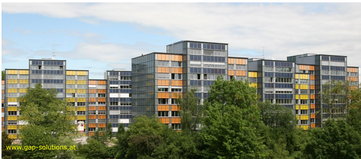
Figure 59. Application of GAP:skin in a building complex (view from South) in Graz, Austria. Source: GAP Solutions.
