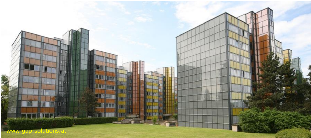
Figure 60. Application of GAP:skin in a building complex (view from North) in Graz, Austria. Source: GAP Solutions.
