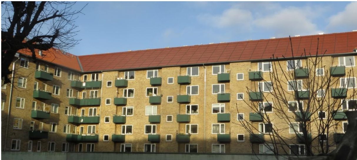
Figure 21. The 52,25 kWp BIPV installation on the roof of “AB Landsdommergaarden” in Copenhagen (Denmark) covers 22 % of the residential electricity consumption. Electricity output: 47.340 kWh during the first year. Estimated CO 2 emissions saved 29.154 kg per year. (Source: Solar Lighting Consultants ApS).
