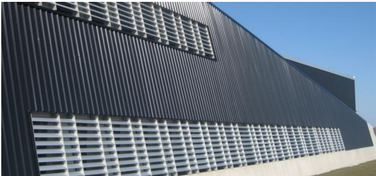
Figure 5. SolarWall installation on the Greater Toronto airport authority building, Canada.
