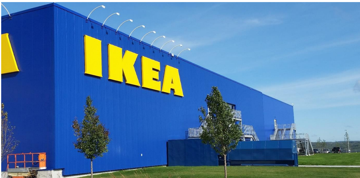
Figure 11. Installation on IKEA, Retail building.
