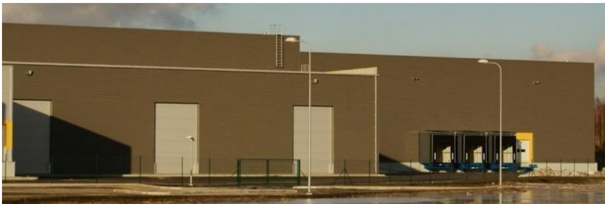
Figure 2. SolarWall installation on a warehouse in Latvia.
