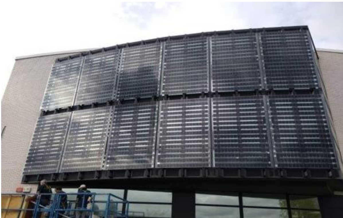
Figure 84. Ventilated façade based on glass-glass back-contact c-Si cells technology BIPV modules developed by Onyx Solar within the framework of PVSITES project at Tecnalia's offices in San Sebastian, Spain.
