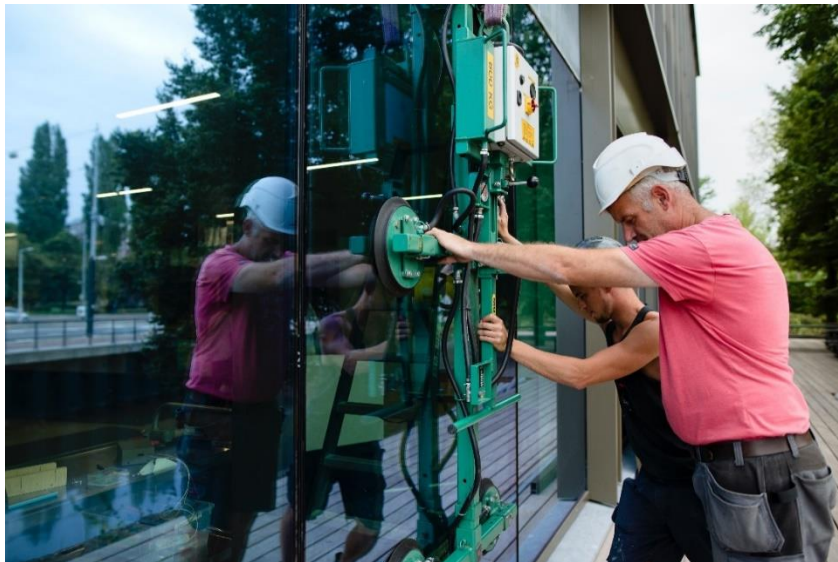
Figure 73. Installation of SmartWindow in EDGE Technologies headquarter in Amsterdam, The Netherlands.
