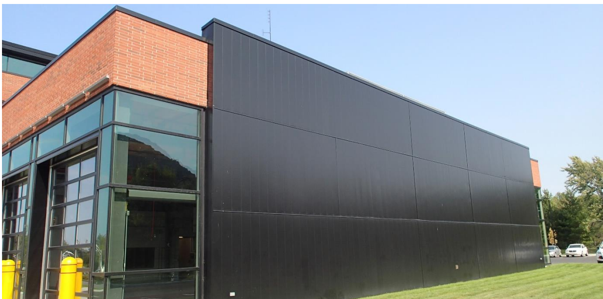
Figure 12. Installation on an emergency services and training facility, Municipal building.
