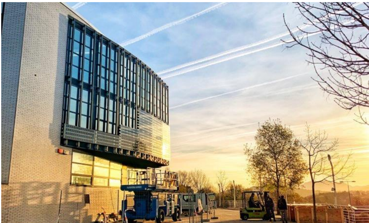
Figure 85. Installation of the ventilated façade based on glass-glass back-contact c-Si cells technology BIPV modules at Tecnalia's offices in San Sebastian, Spain.
