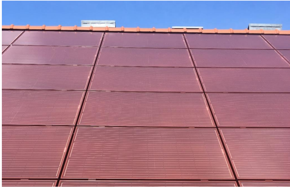
Figure 20. SUNERG X – Color monocrystalline modules in roof application, colour of the module: chestnut brown (RAL 8015) (Source: Solar Lightning Consultants ApS - Architect Martin Dietz (C)).
