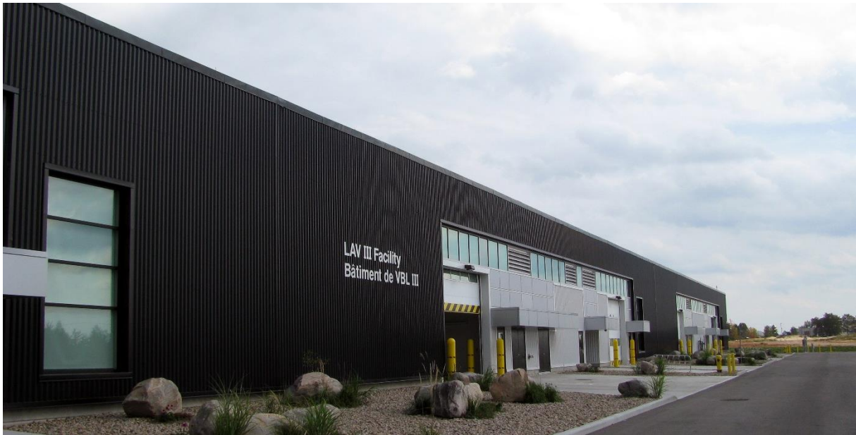
Figure 13. Installation on Light Armoured Vehicle Maintenance Facility, Military building.
