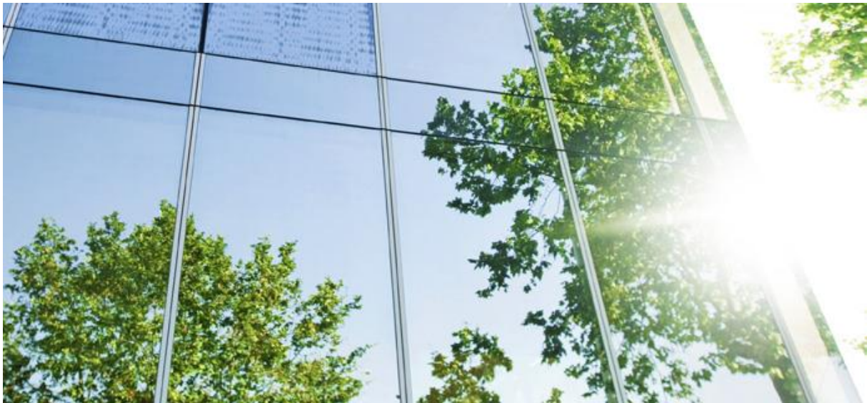
Figure 51. LCWs viewed from the external environment.
