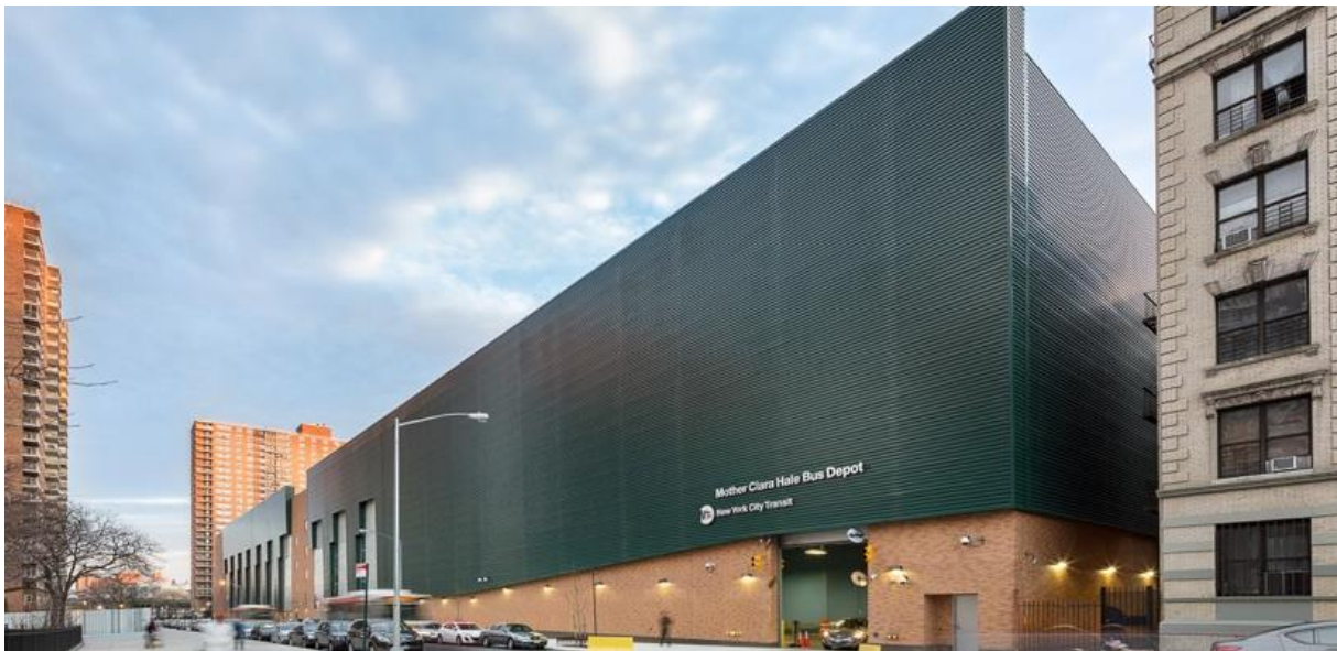
Figure 4. Dark green SolarWall collectors on three walls of a bus garage, New York City.
