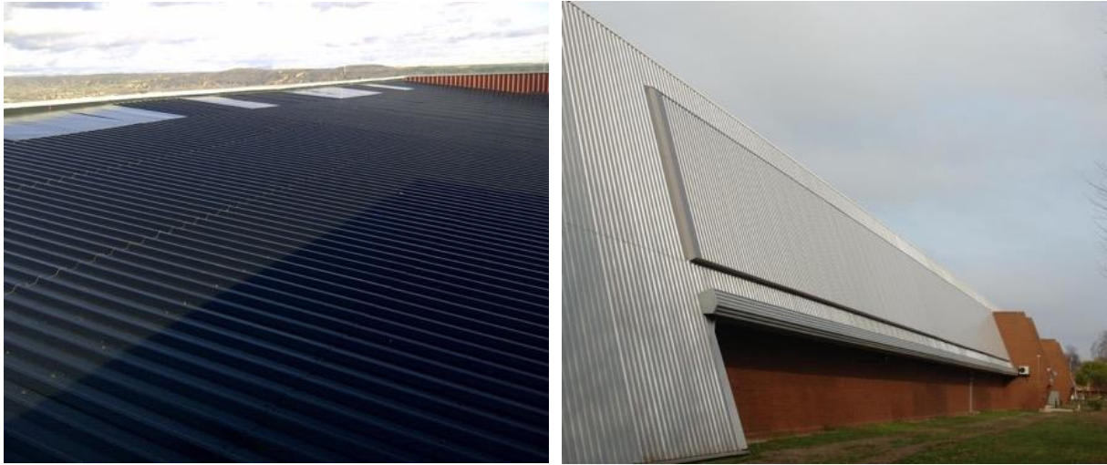
Figure 3. Roof-mounted SolarWall on a hospital in Spain (left) and Jaguar/Land Rover training centre in England with grey collectors to match the colour of the main wall (right).
