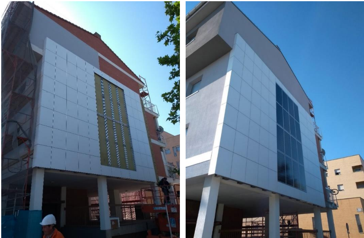
Figure 34. Installation of BHFS in a demo-building in Zaragoza, Spain (Source: ACCIONA Construcción).
