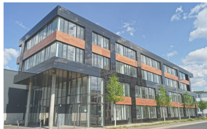
Figure 3: Impressions of solar systems in Berlin Adlershof (photos: Margarethe Korolkow).
