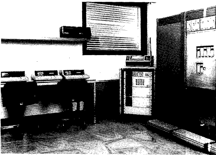
Figure 2.5.5. J.R.C. outdoor test field: data acquisition system for collector efficiency test, DHW monitoring and meteorological data.
