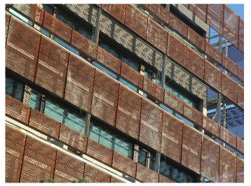
Figure 1. South view of the double skin micropeforated façade of IDOM Headquarter in Madrid. This façade is perhaps its most distinctive sign. The façade, which was designed to reduce overheating, provides also some glare protection if combined with roller shades.
