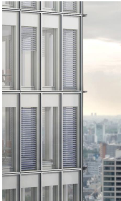
Visual impression of solar thermal venetian blinds, Arkol project. © IBK2
