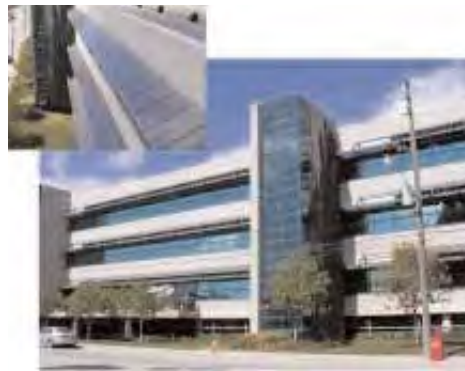
The Toronto Hydro Energy Services 35kWatt PV façade.
