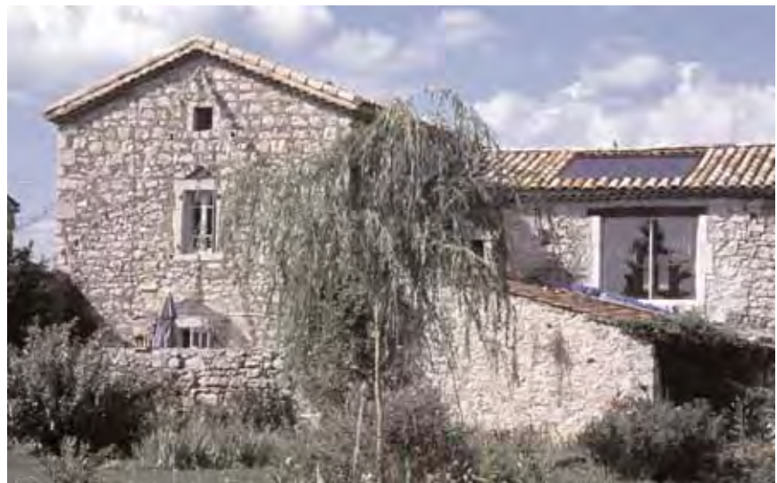
Figure 2. Single-family solar heater at LUSSAS (Ardèche, centre of France), with roof-integrated collectors
