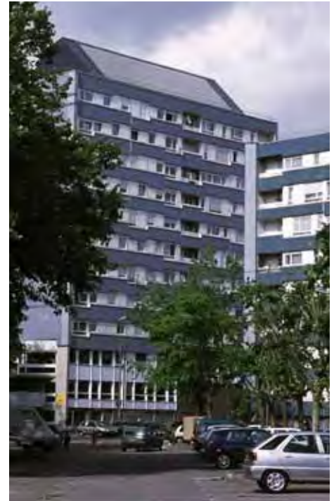
Figure 1. A medium-scale SDHW plant (180 m 2 ) for the health center at BRIANCON (Hautes-Alpes).
