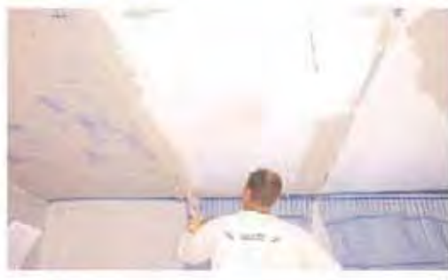
Figure 3. Micro-encapsulated PCM and plastic capillary mats for “LowEx” heating and cooling in walls and ceilings.
