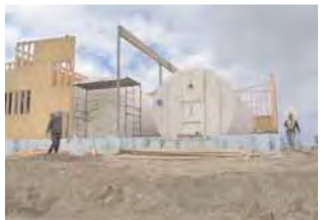
Installation of Short-term Storage Tanks in the Energy Centre.
