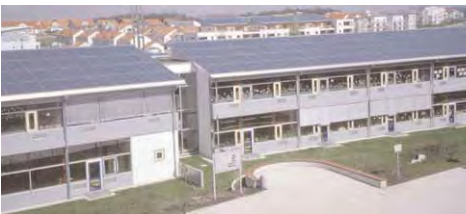
Figure 2. Solar Plant Neckarsulm-Amorbach in Phase II (expanded 6,300 m 2 solar collector roof and a 65,000 m 2 duct storage) and operating since 1997.
