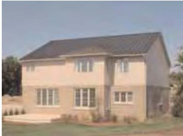
Residential System utilizing roof-integrated amorphous PV technology.
