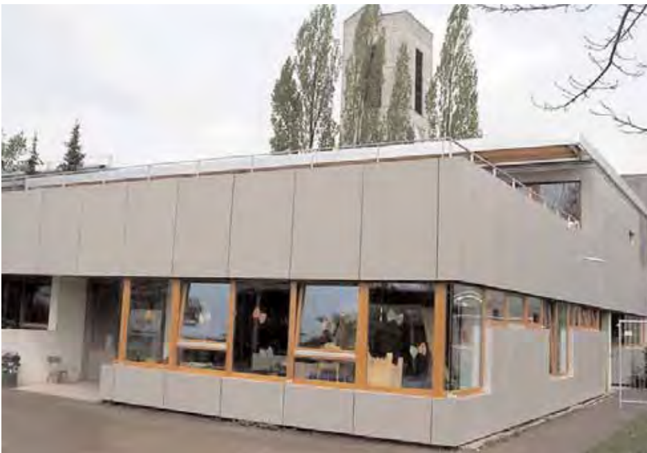
Figure 5. Renovation of the Kindergarten with vacuum panels in the facades and ground floor (photo by IBP)
