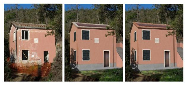
Figure 128: Simulation of a new coloured PV roof (almost integral) on slate or on tiles. A) the current state, b) the new roof inserted on slates, c) the new roof inserted on tiles (FAI).
