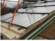
Figure 32: PVT solar modules. © D. Studer, Studer Architekten
