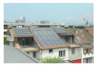
Figure 15: Roof with solar thermal and PV, Viridén + Partner AG Architects, © Nina Mann
