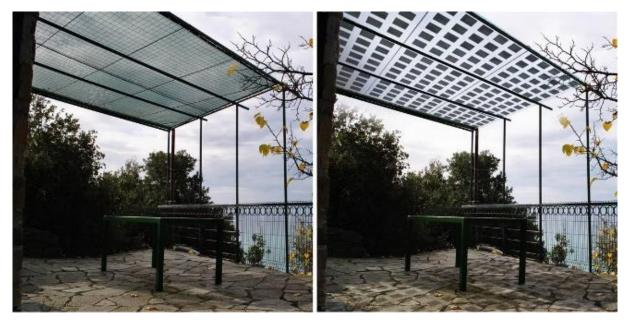
Figure 125: Monestiroli, photo-simulation of a compatible intervention. On the left, current state, on the right, the use of transparent PV cells
