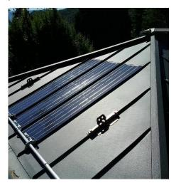
Figure 140: The PV panel applied on the metal roof, Valentina Carì Progetto Serr@
