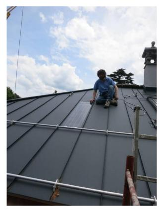
Figure 96: BIPV roof construction, ©Valentina Carì, Progetto Serr@
