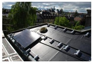
Figure 100: Single family House, Bern. Installation of PVT+PV panels, © M. Hutterli
