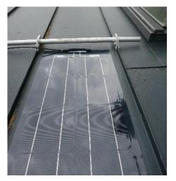
Figure 141: The PV panel applied on the metal roof and connection cables, © Valentina Carì Progetto serr@
