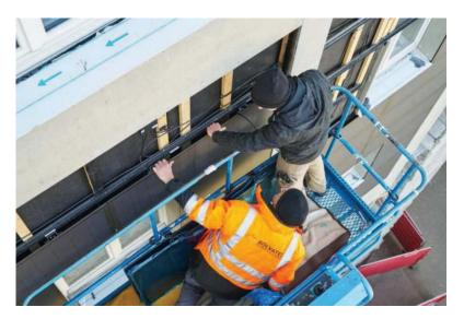
Figure 138: Installation of PV modules on back rails, . Picture: © Martin Zeller
