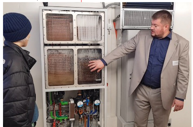
▲ The Green Chiller Association offered a tour around a mobile sorption classroom. The completely open absorption cooling system makes it possible to explain the technology clearly and illustrate various operating states. Christian Kemmerzell, Managing Director of EAW Energieanlagenbau, demonstrates the unique system. (Photo: Bärbel Epp)
