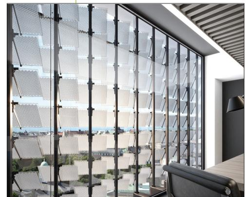
▲ **Figure 1. Examples of solar envelope systems described in SHC Task 56 report, State-of-the-art and SWOT analysis of building integrated solar envelope systems. On the left, Kromatix BIPV panels (photovoltaics, Swissinso). On the right, Lumiduct (photovoltaics and shading system, TUE).**
