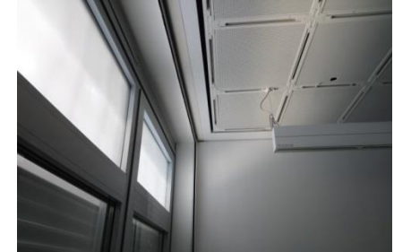
2 test façades with test cells
