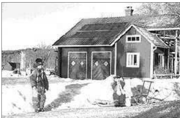
Solar combisystem for a single-family house in Sweden. (Source: SERC)
