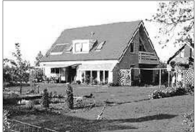
This French house uses a solar floor heating system to meet hourly and overnight variations in the solar energy supply. (Source: Clipsol)
